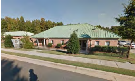
Street views of existing buildings
